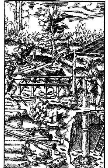
Figure 51: Manually driven piston pump.
