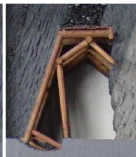
Figure 34: Combined timbering with polygon support.
