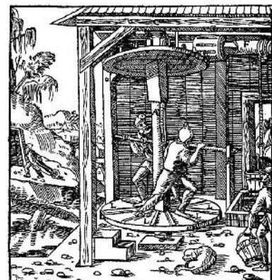
Figure 47: Winch with thread mill.
