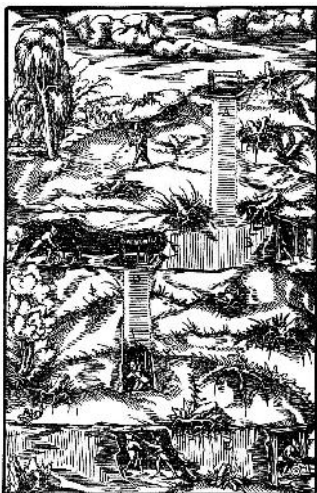
Figure 15: Cross-drifts and shafts. Shafts (A, D), cross-drift (BC), Adit (D), adit entrance (E).
