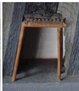
Figure 33: Combined timbering with polygon support.
