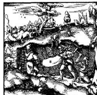
Figure 21: Ventilation with waved sheets.
