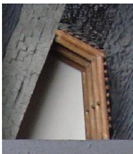
Figure 31: Half khûzan timbering.
