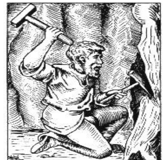
Figure 12: Cutting with chisel and mallet.
