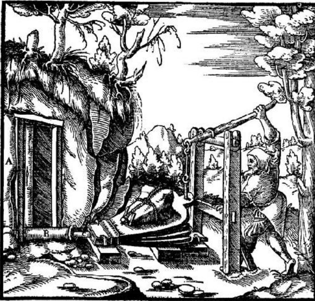
Figure 24: Ventilation by usage of bellows and air ducts.
